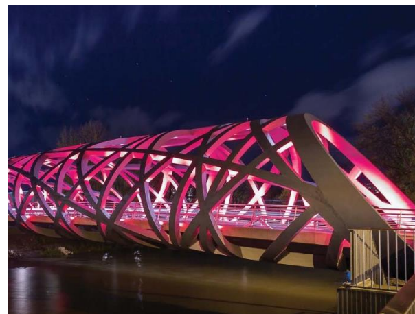
HANS WILSDORF BRIDGE Geneva, Switzerland
